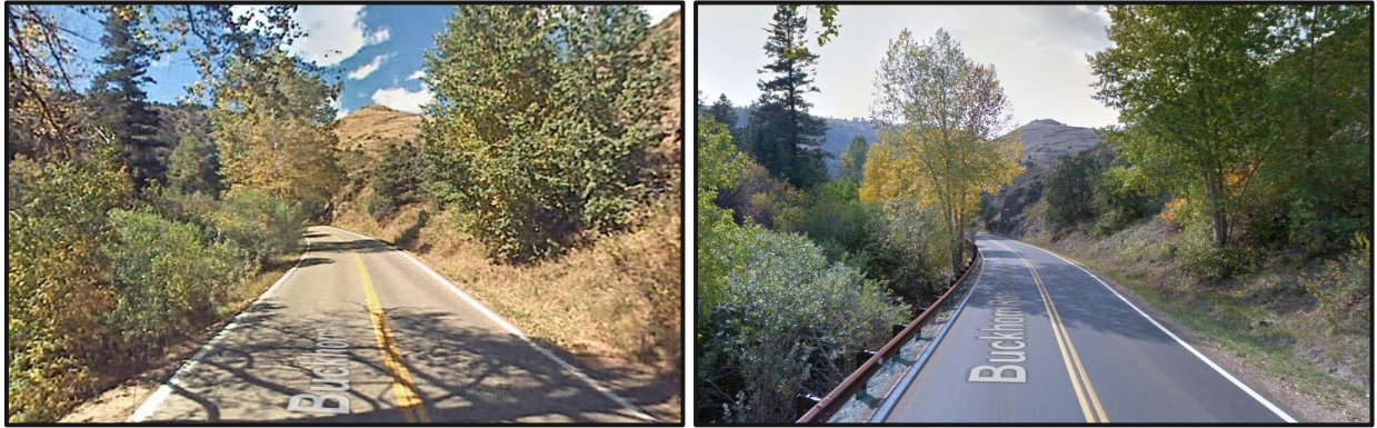
LCR 27 (Buckhorn Road) – Before (left) and After (right) improvements
