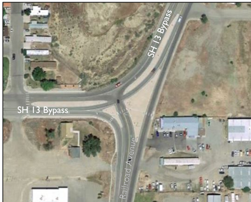
Railroad Avenue & SH 13 Bypass in Garfield, Colorado
