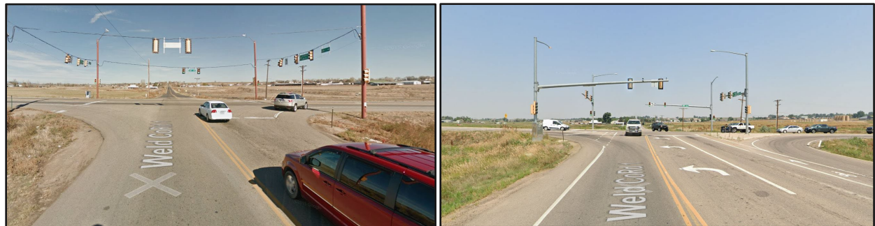
WCR 1 – Facing North – Before (left) and After (right) Improvements
