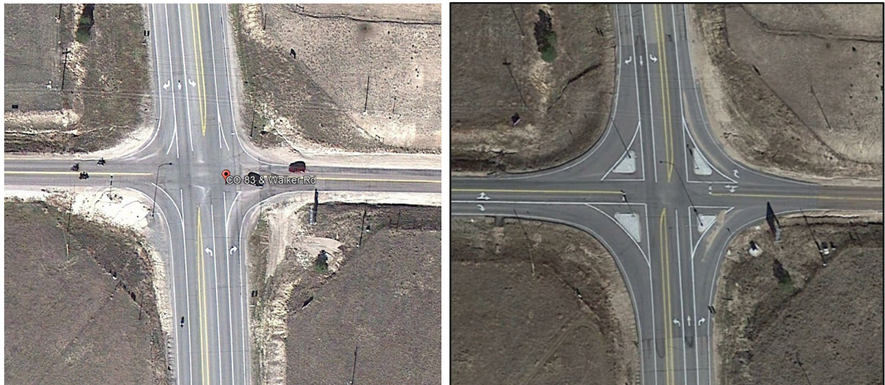
SH 83 & Walker Road before (left) and after (right) improvements
