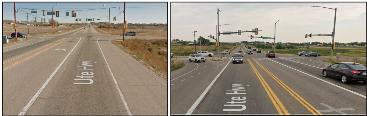
SH 66 – Facing East – Before (left) and After (right) improvements
