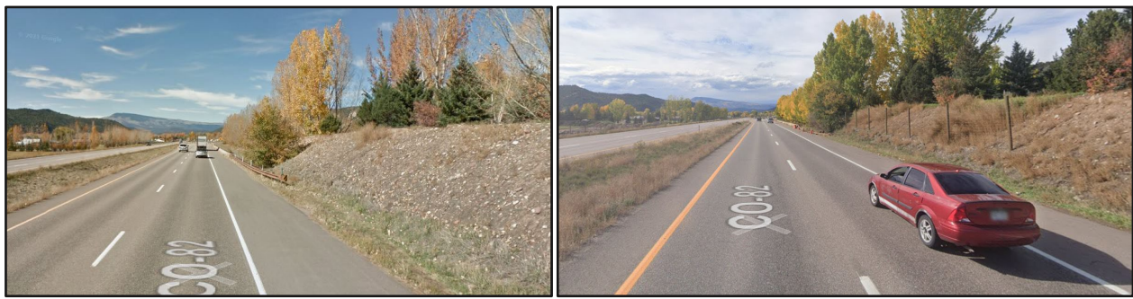
SH 82 – Southbound – Before (Left) and After (right) improvements
