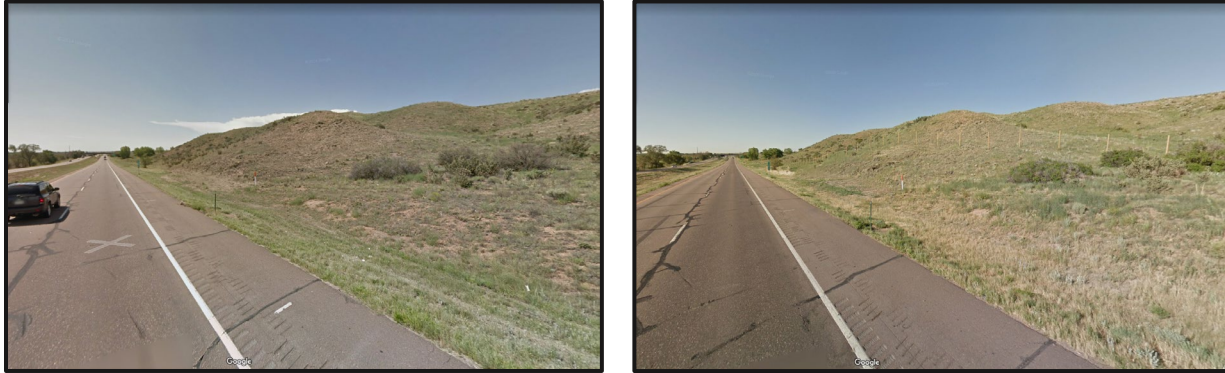
I-25 – Southbound – Before (Left) and After (right) improvements
