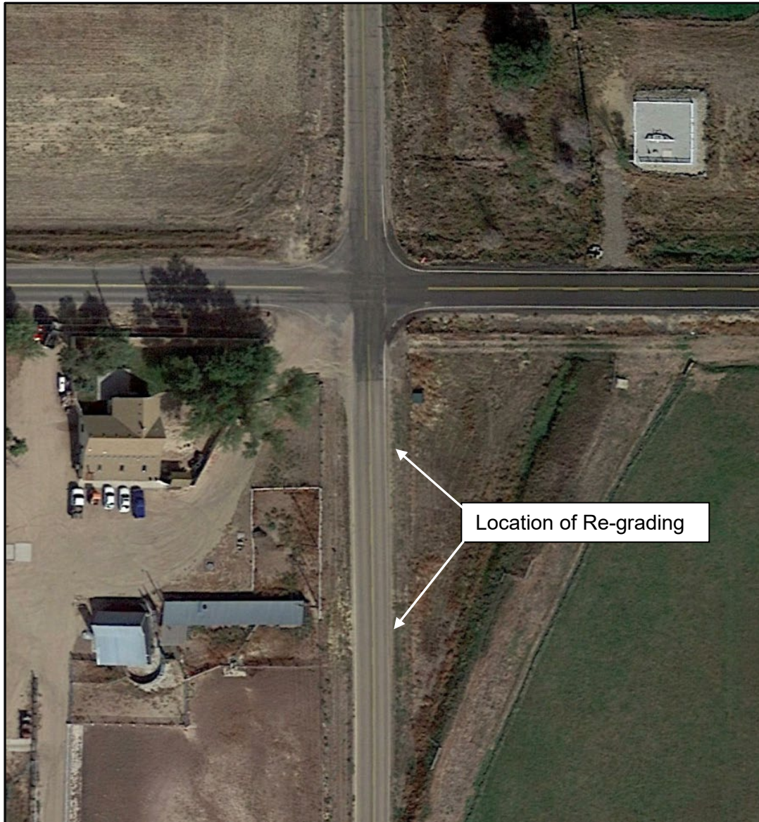
Figure 1: CR 17 at CR 34 in Weld County
