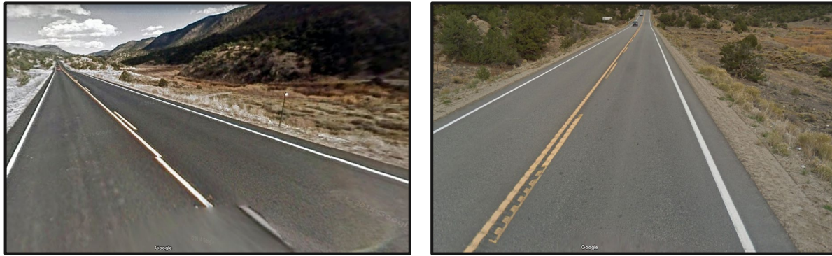
US 24 – Facing North – Before (left) and After (right) improvements
