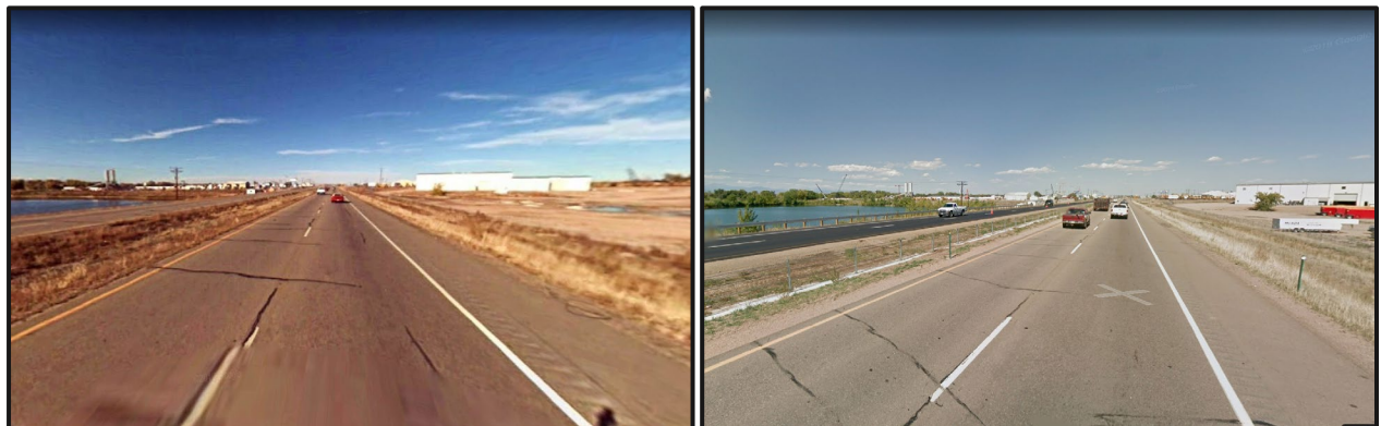
US 85– Facing North – Before (Left) and After (right) improvements
