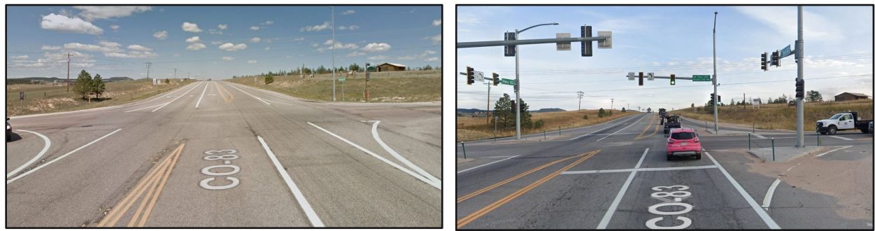
SH 83 & Walker Rd – northbound – Before (left) and After (right) improvements
