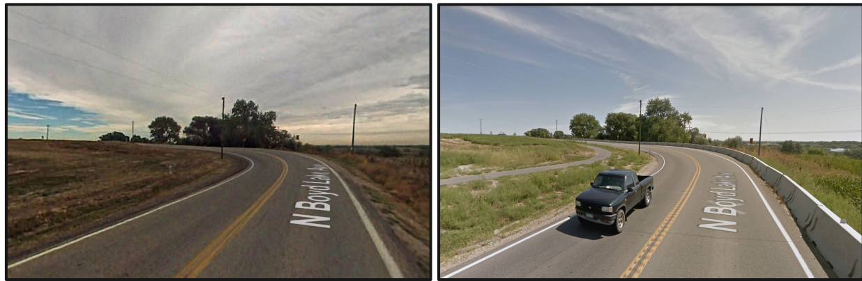
5 th Street & Boyd Lake Avenue – Facing Northeast – Before (left) and After (right) improvements
