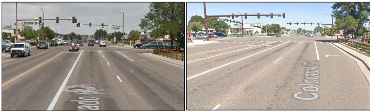
Colorado Blvd – Facing North – Before (left) and After (right) improvements
