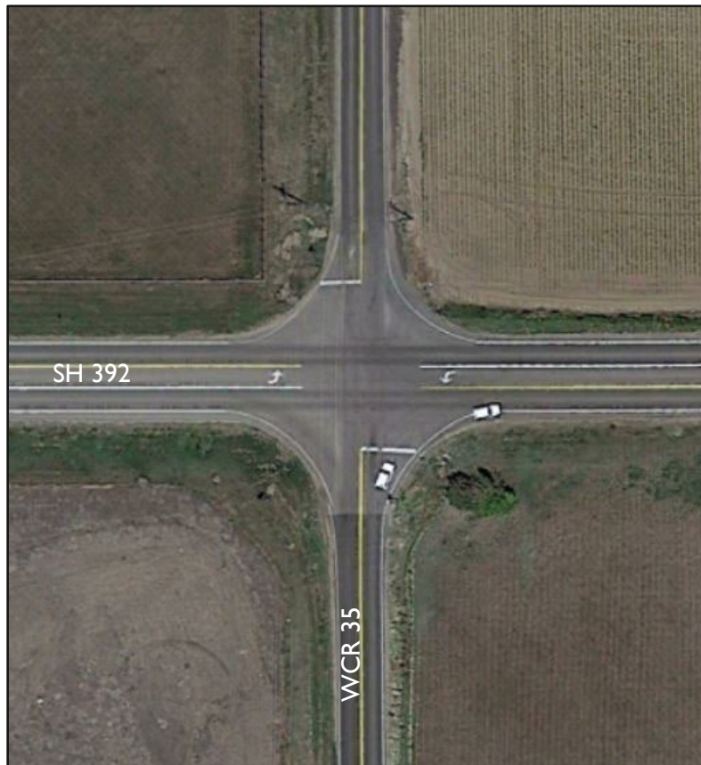
SH 392 & WCR 35 in Weld County, Colorado
