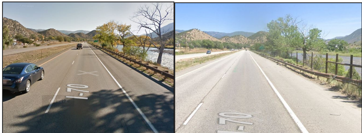
I-70 – Southbound – Before (Left) and After (right) improvements
