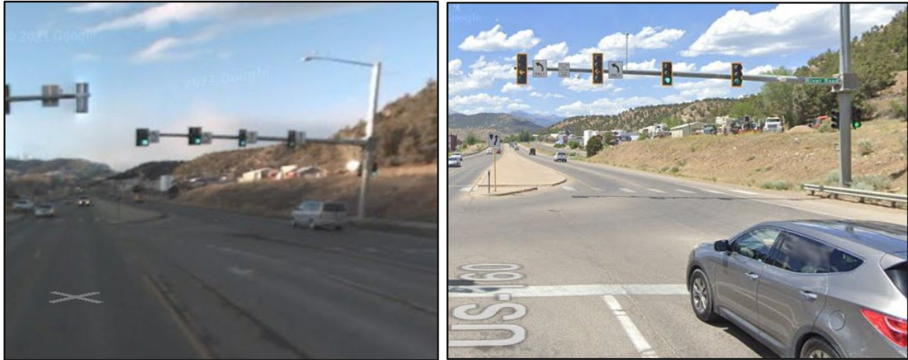
US 160 & River Rd – Northbound Before (left) and After (right) improvements
